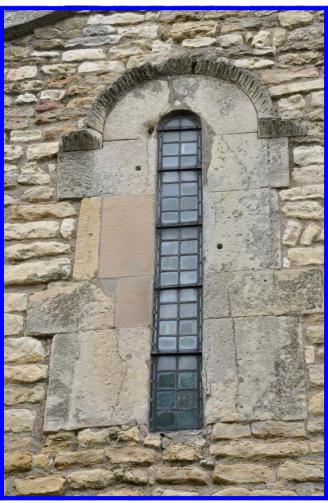
transept. Note the hood worked with palmette decoration (this matches the work on the nave crossing archway.) The dimensions of the aperture of this window are approximately 6ft 6in tall x 10in. wide. Its sill is approx. 13ft 6in. above the lowest order of the plinth. Thickness of the wall is 2ft 6in. This window, dating to the 'upper work' (after the fire), can reasonably be assigned to the work of Eadnoth I in the first half of the 11th century. (source: H.Taylor)
