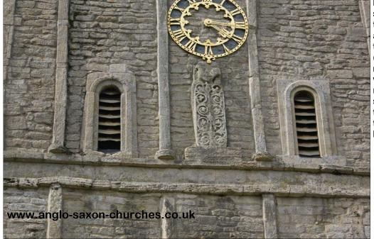
blocked up. It may be noted that the first stage has rather random quoin stones but the second stage has long-and-short work and is cut back to allow a plaster covering to be run up against the upstanding edge (see picture). This should be borne in mind when viewing the windows which would have shown as the upstanding 'rib' running around the window surrounded by plaster rendering covering the main surface of the walling. It seems there are two stages/dates of building here.
